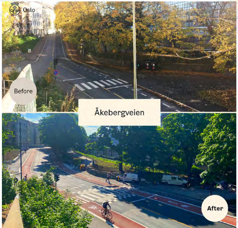
View of the street Åkebergveien in Oslo, Norway. Parking was removed to make room for a temporary bike lane going uphill before the street was rebuilt.
