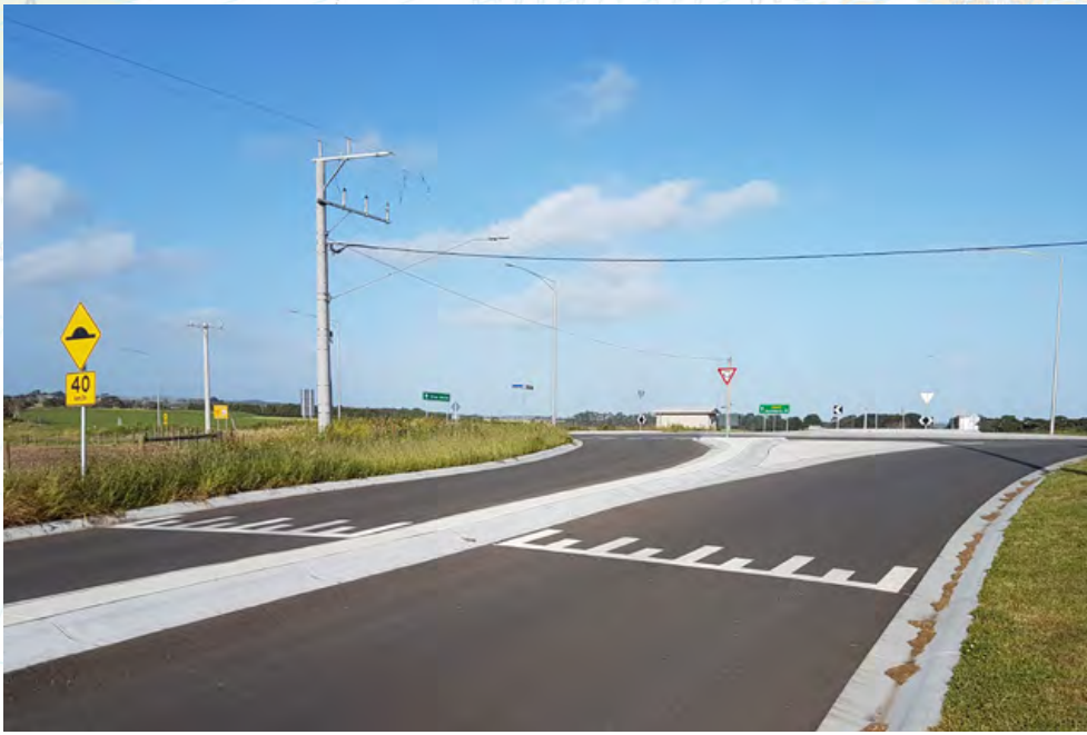
This high-speed roundabout in Victoria, Australia, uses a raised platform to manage speed.
