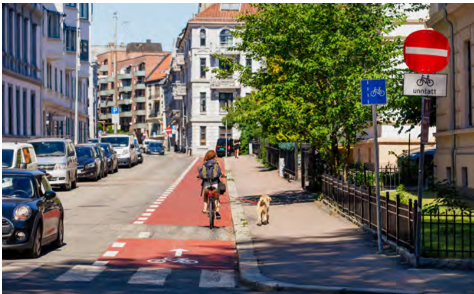
Shown here is an example of a counterflow bike lane in a one-way street in Oslo. Motorized traffic volumes are typically low in one-way streets, reducing the number of interactions that may end in crashes.
