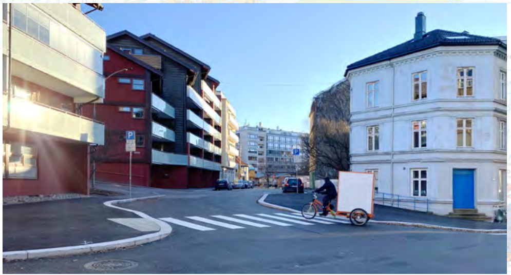
This narrowing of an intersection forces a speed reduction for motorized traffic that are about to turn. This improves a driver's and cyclist's ability to notice one another and interact in a safe manner. Narrowing intersections also reduce crossing distances for pedestrians and the amount of time they are exposed to motorized traffic.
